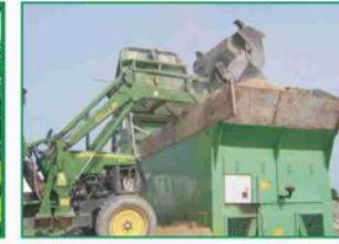
Material handling at Batching plant
